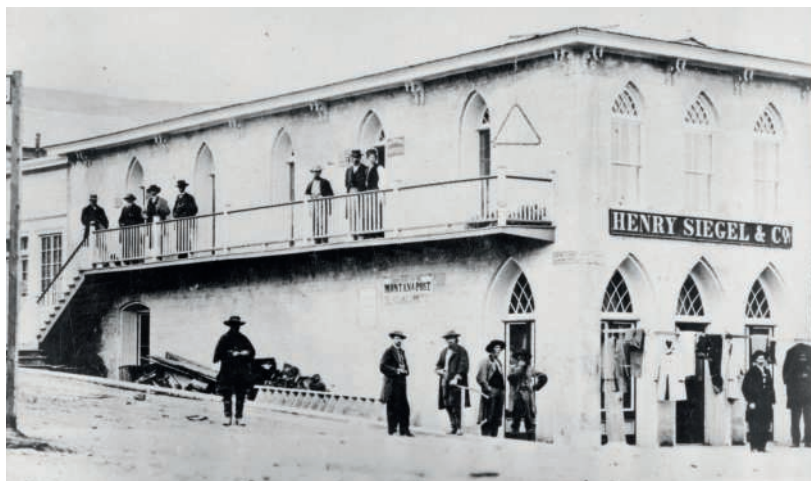
Historic American Buildings Survey Courtesy of Historical Society of Montana, Southwest corner of Wallace & Jackson Streets, Virginia City, Madison County, MT. Courtesy of Prints and Photographs Division, Library of Congress (HABS MONT,29-VIRG,2-2).
